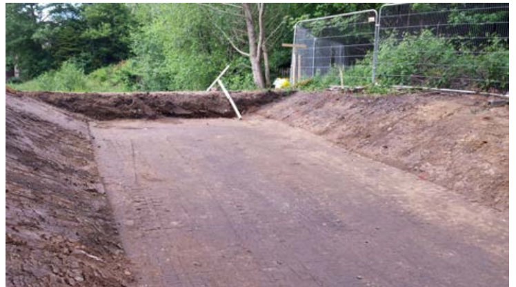
Picture 6 - Spillway under construction at Viaduct Pond.
